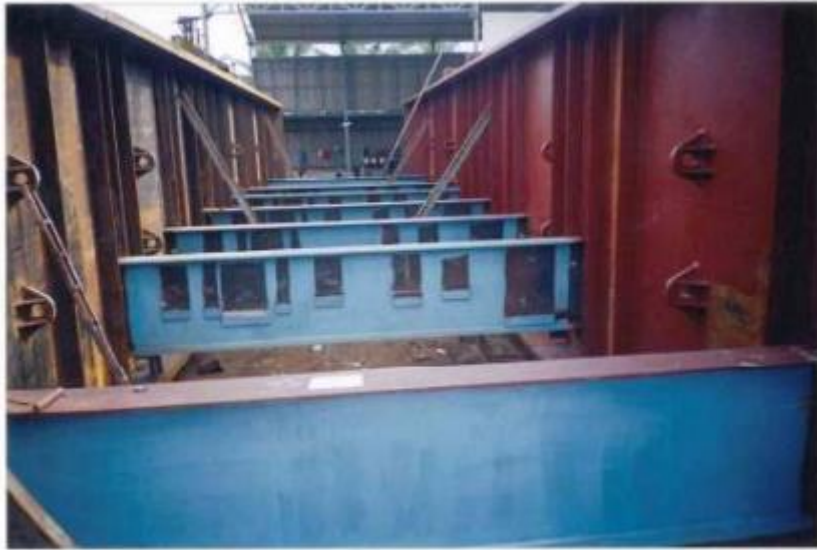
CEILING GIRDER ASSY PROJECT: SHIMADRI (NTPC) WT: 250 MT
